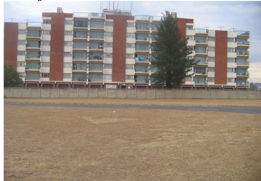
Arbor Heights lift to be refurbished
